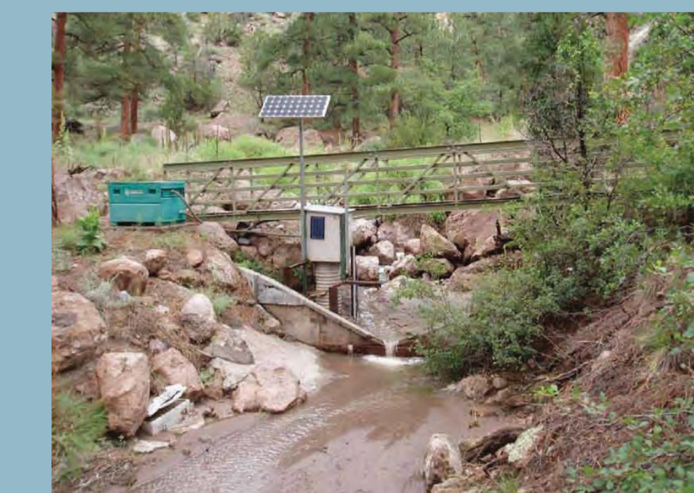
Typical surface water monitoring gage station
