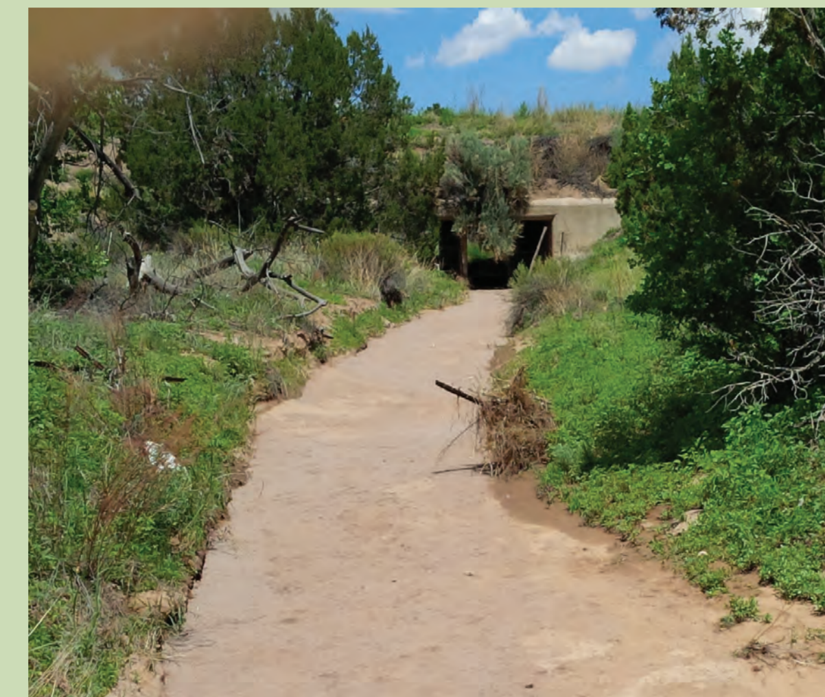
Storm flow in typical ephemeral channel
